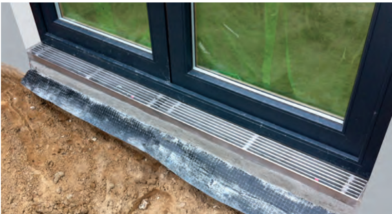
The one-piece channel is manufactured to fit the reveal
