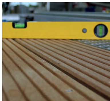
Check the installation height
