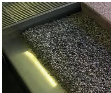
Inserting the gavel and subsequent installation the block pavement
