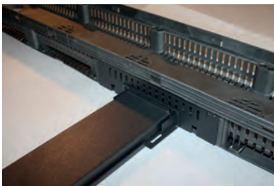
Position the reveal drain-off element
