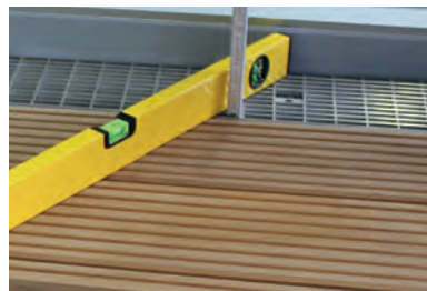
Fitting of the wood terrace channel
