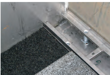
Channel system loosely installed
