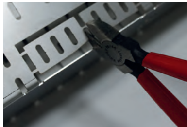
Opening the branch channel connection
