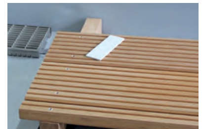
If necessary, place material below the channel body
