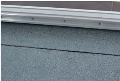
Connection of a bitumen-based sealing ring with a wedge
